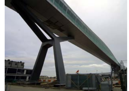
Figure 1: Exterior view of bridge.
